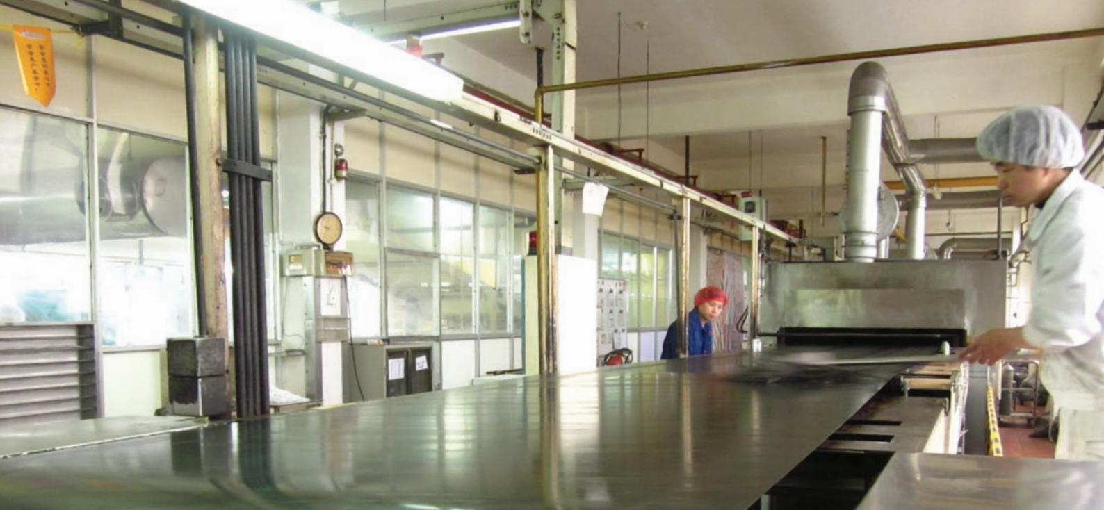
Installing IPCO's solid steel belt
